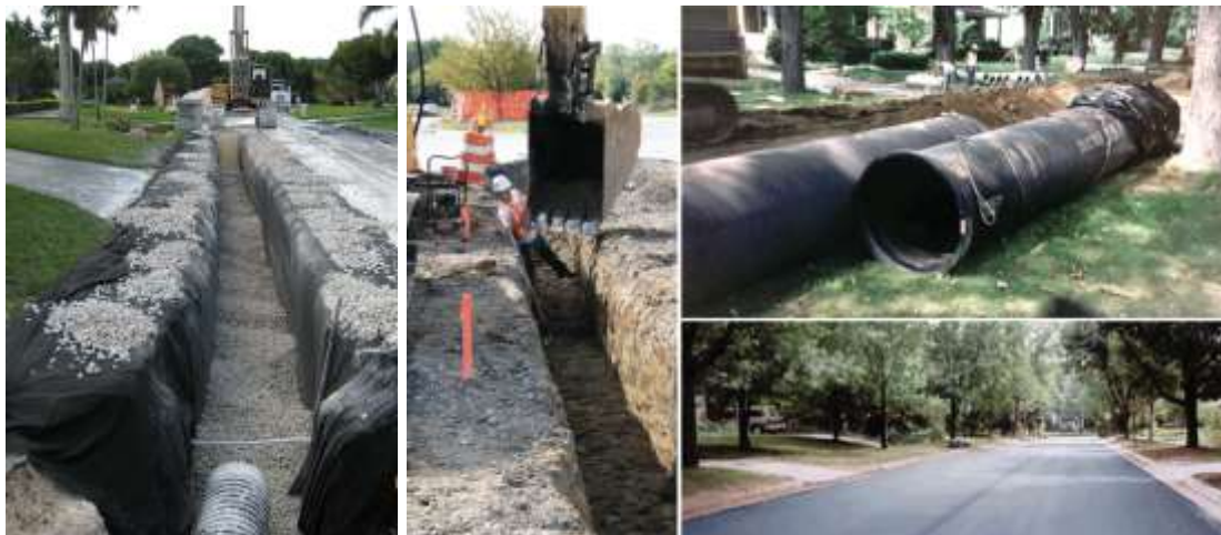
Figure 6.12 – Exfiltration Trench
