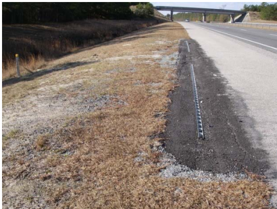
Figure 4. Edge-of-pavement slot drain.
