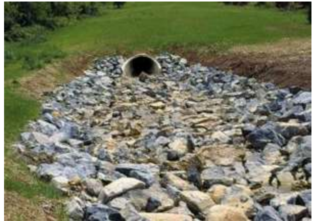
Figure 10.6 – Stone Check Dams in Swale and Stone Outlet Trap
