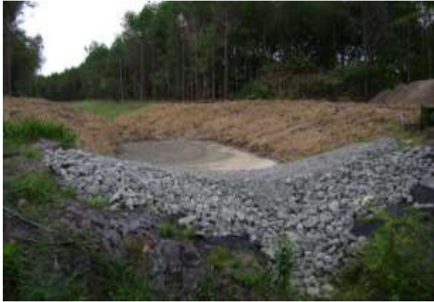
Figure 10.4 – Sediment Trap & Spillway
