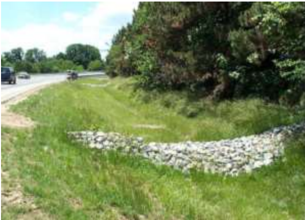
Figure 10.6 – Stone Check Dams in Swale and Stone Outlet Trap
