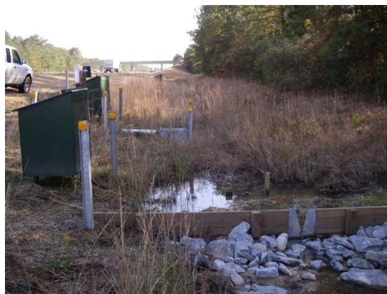
Figure 8. Outlet structure for swales.
