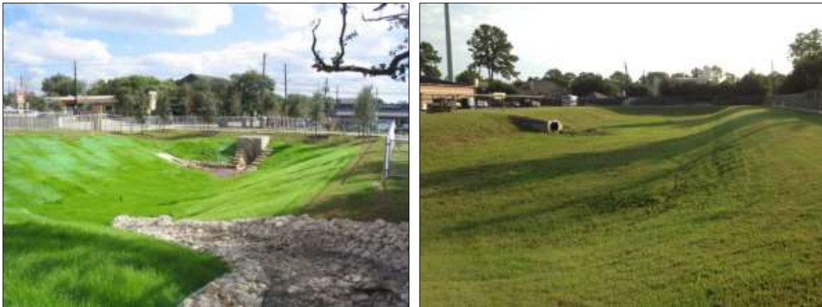
Figure 6.20 – Typical Dry Retention Pond
