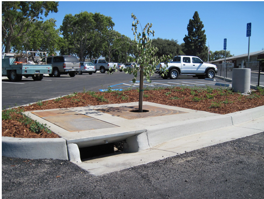
Figure 12 - Newly Installed Urban Green BioFilter
