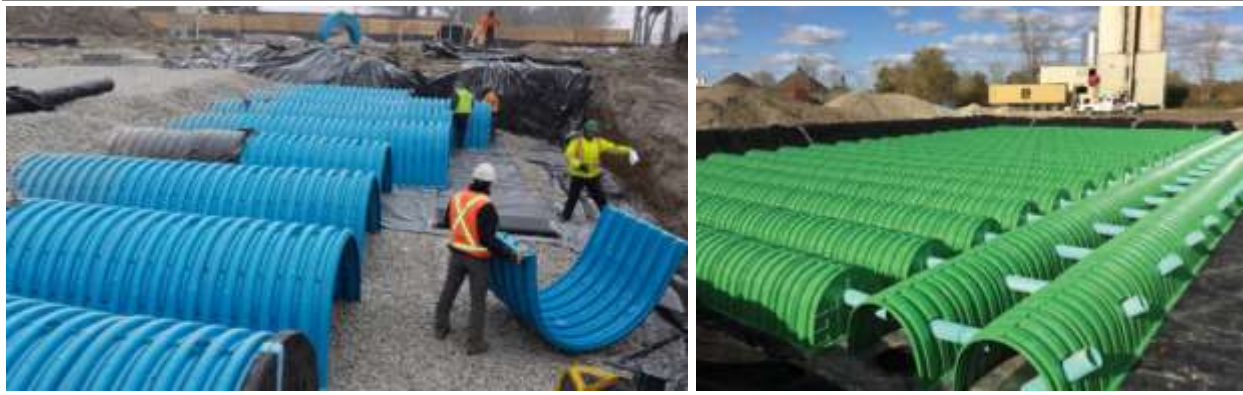
Figure 6.22 – Stormwater Chambers
