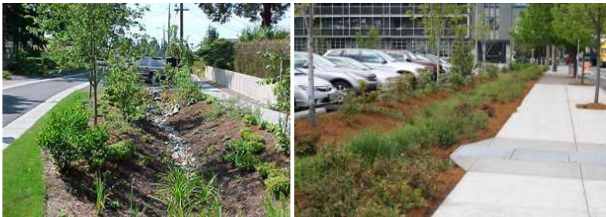
Figure 6.6 – Vegetated Swale in a Residential Area and a Parking Lot
