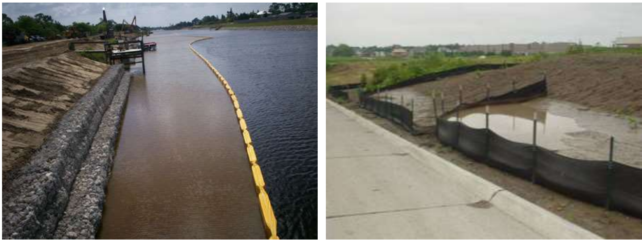
Figure 10.3 – Stacked Turbidity Barrier or Silt Fence (c)
