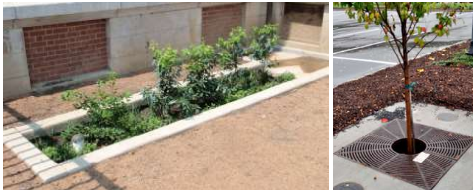
Figure 6.4 – Infiltration Planter and Tree Box
