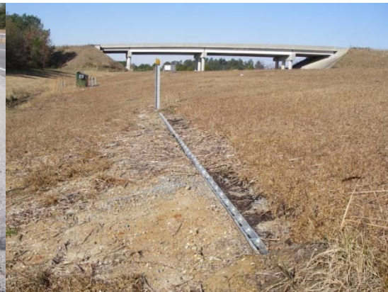
Figure 5. Downslope edge of filter strip slot drain.
