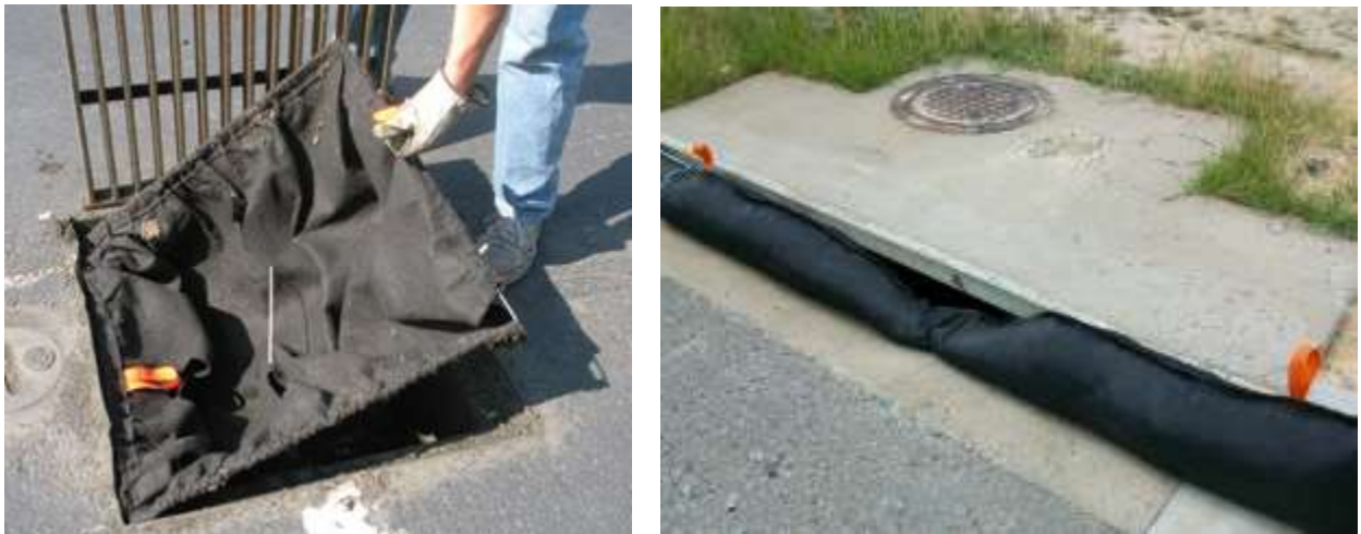
Figure 10.2 – Storm Drain Inlet Protection (b)
