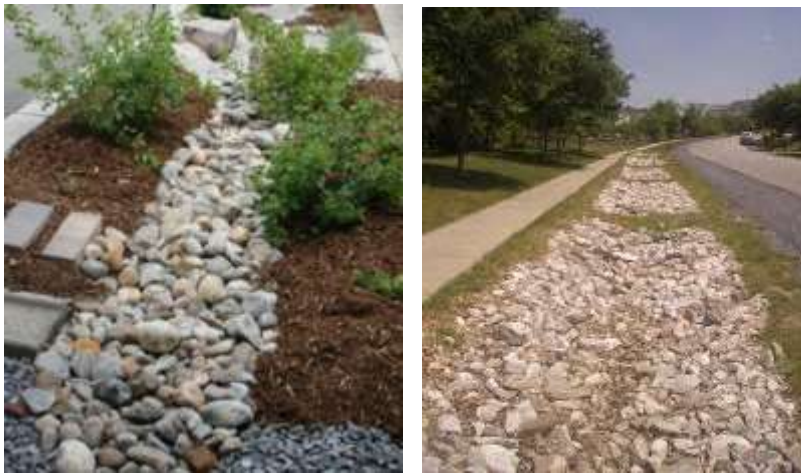
Figure 6.10 – Infiltration Trench
