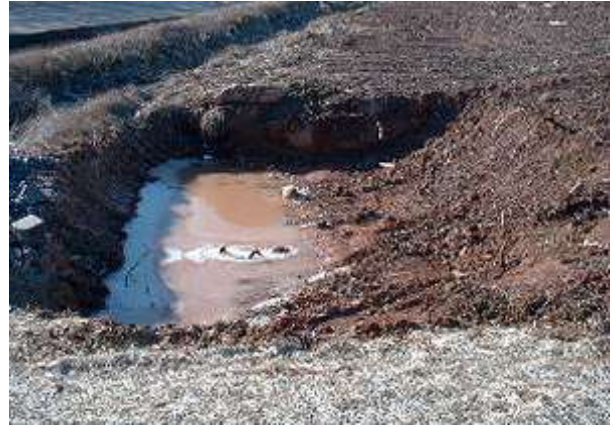
Figure 10.4 – Sediment Trap & Spillway
