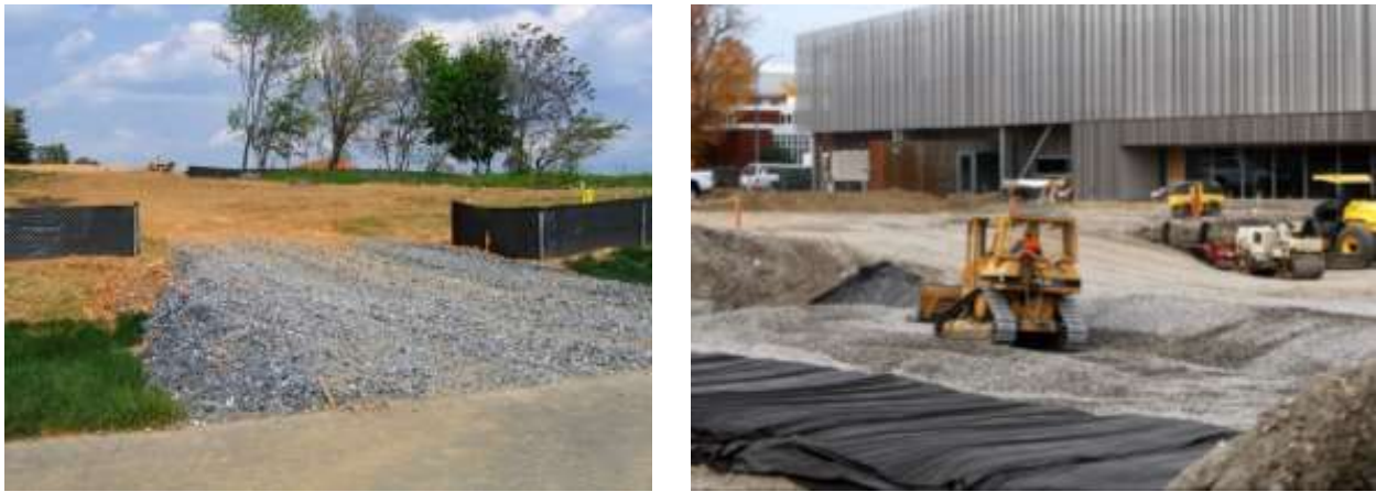
Figure 10.1 – Temporary Gravel Construction Entrance & Exit (a)
